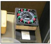
If heating times do not match building occupancy, energy is wasted. Matching heating times to occupancy will reduce energy usage and costs and enhance comfort levels. We recommend reviewing night storage controls.
