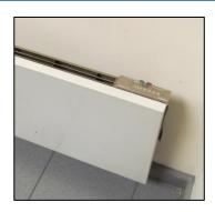
The office heating is a mixture of night storage heaters and electric wall-mounted fan convector heaters. The night storage heaters in the office are manually set by Mark to maximise heat output and seasonally adjusted.
