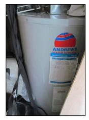
Your hot water boiler in the upstairs changing room is permanently switched on and heating water 24 hours a day 365 days a year. The boiler is rated at 9.5kW and will use about 5kW a day to heat the water.
